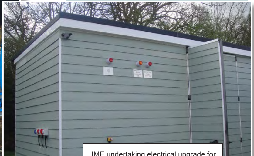
IME undertaking electrical upgrade for IGAS Ltd at Larkwhistle Farm 2012
